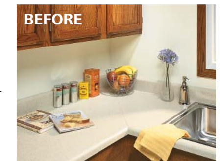
Although completely functional, this outdated post-formed countertop made for a bland kitchen.
